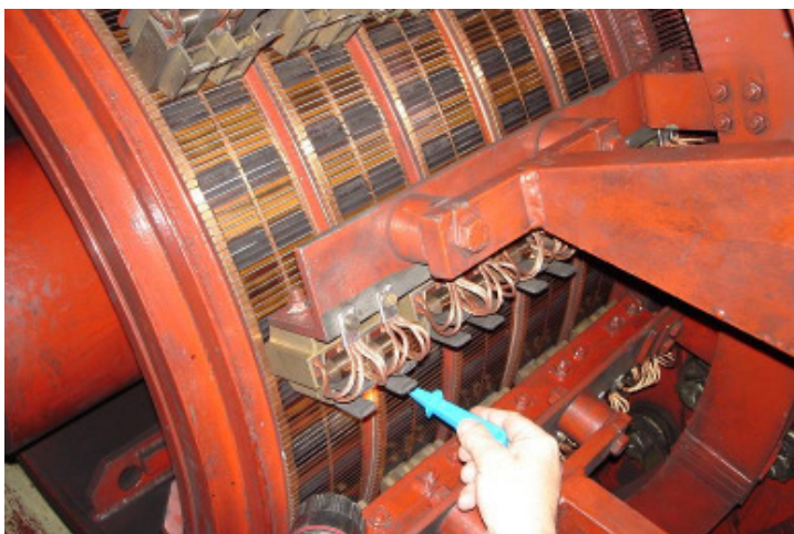
Broken commutator lead
