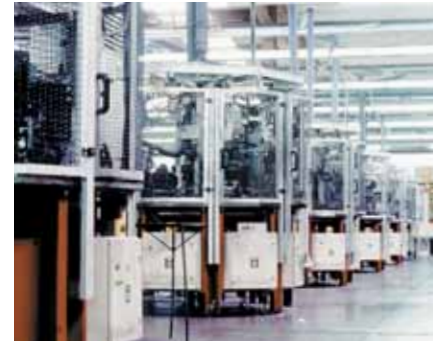
production hall with modular automatic rotary tables
